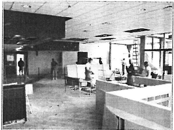
Photo courtesy of Mark Chandler Felicita's during its 270,000 dollar renovation.
